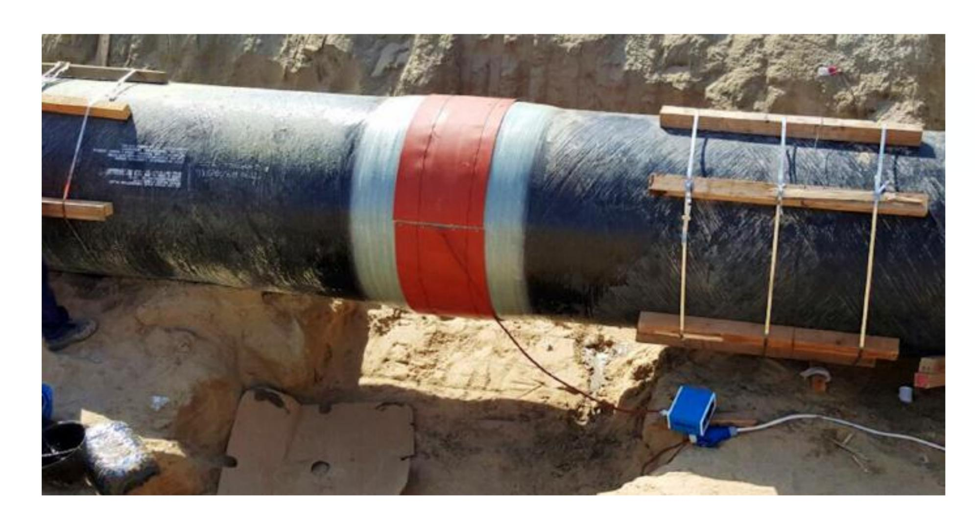
Adjust The Temperature of the Built In Regulator on Heating Blanket to the required Heat. In the following example of How to wrap (Page 5 and Page 6 for Wrong vs Right), we set the temperate to 92.5 °C
